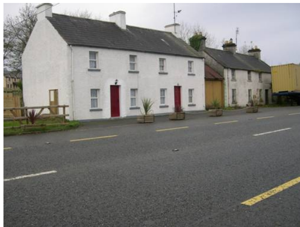
Plate 5 CHC 09 – early 19 th century structures, Toberscanavan village, Mullaghnabreena Td
