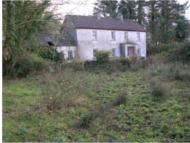
CHC 81 – early-mid 19 th century structure, Drumderry Td
