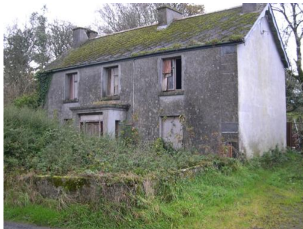
Plate 75 CHC 84 – early 19 th century structure, Drumderry Td
