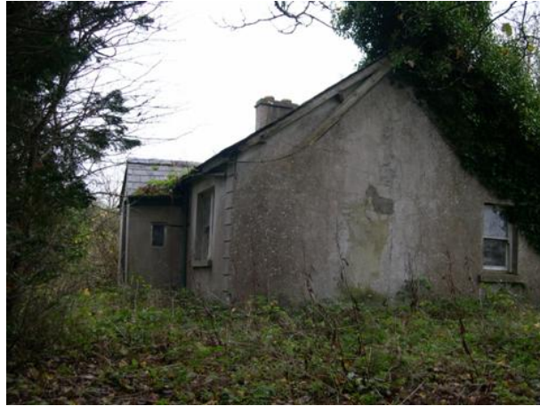
Plate 25 CHC 32 – 19 th /20 th century structure, Doorly Td
