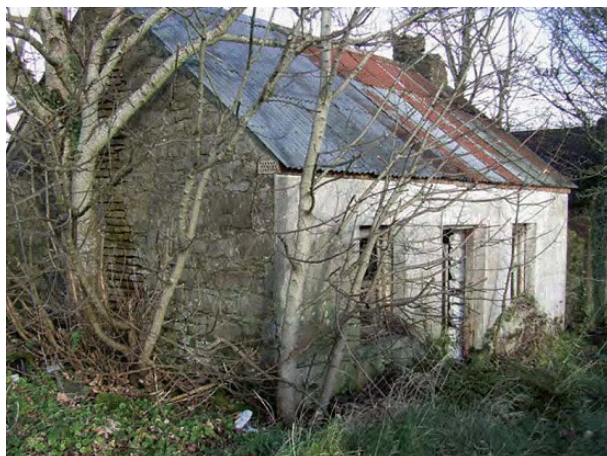
Plate 30 CHC 38- 19 th century structure 'school', Knocknagroagh Td.
