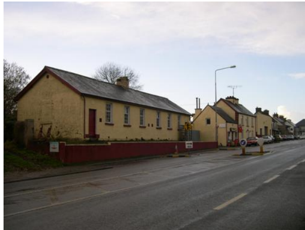
Plate 82 CHC 91 – Protected structure ‘Former Castlebaldwin National School’, Draft RPS 84, Cloghoge Upper Td
