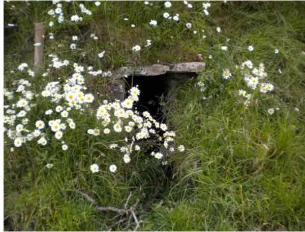
Plate 37 CHC 46 Stone-lined culvert, Drumfin Td.
